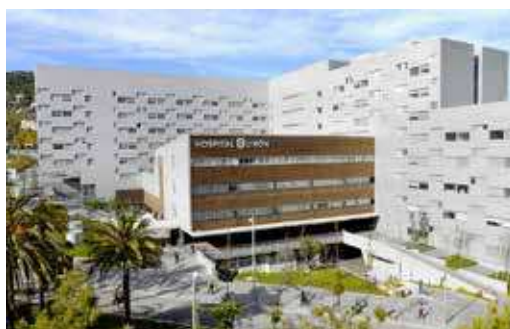
HOSPITAL QUIRÓN BARCELONA
