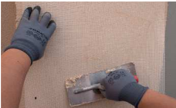
7. Colocar la malla RG-116 Isolxtrem System.
