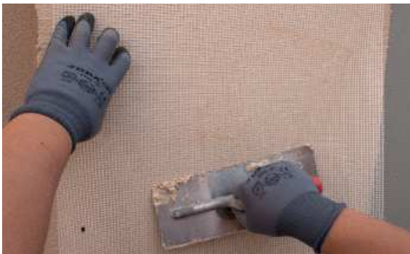
7. Colocar la malla RG-116 Isolxtrem System.
