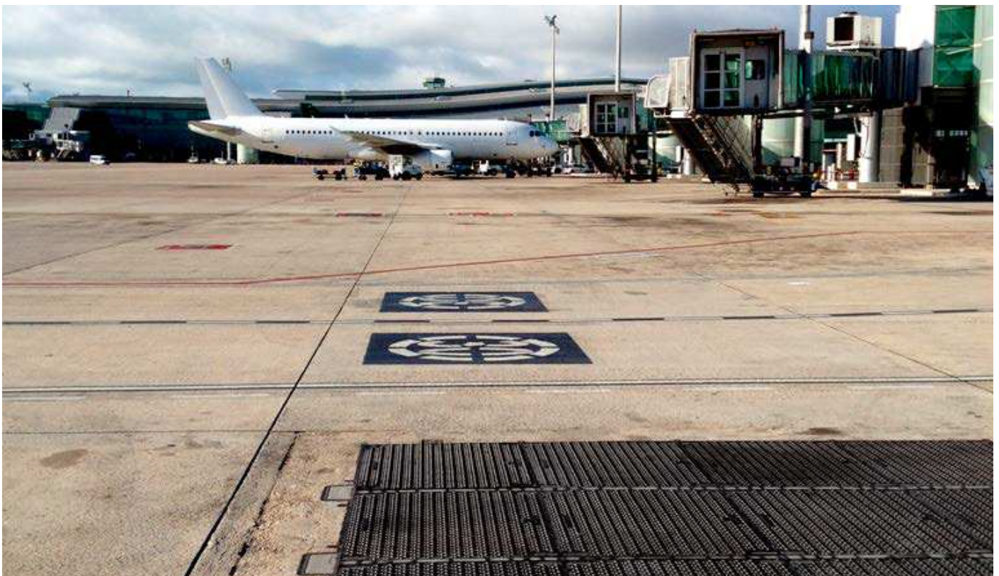
Barcelona International Airport - Barcelona, Spain
