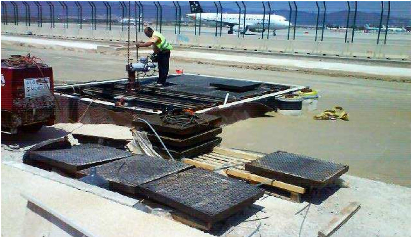
Barcelona International Airport - Barcelona, Spain
